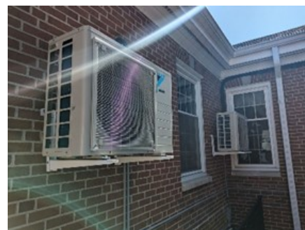
Outdoor Heat Pump With new Masonry & Matching Bricks
