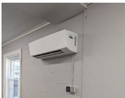
Indoor Highboy Unit and Thermostat With New Drywall & Painting
